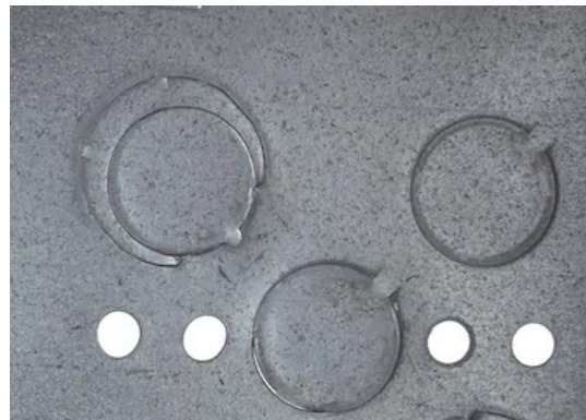
Example of 1/2" and 1/2" & 3/4" Combination Knockouts
