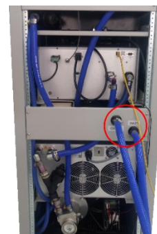
Figure 4: Supply and return hose connections
